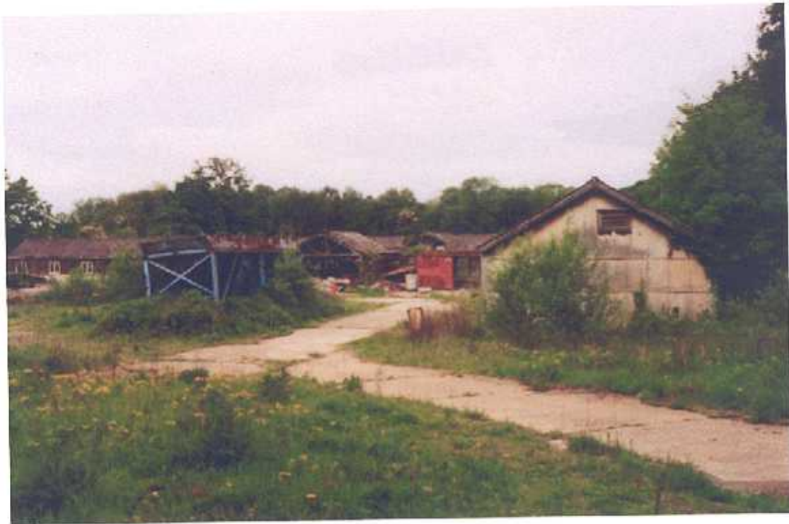
Plate 1: General view of site looking south
