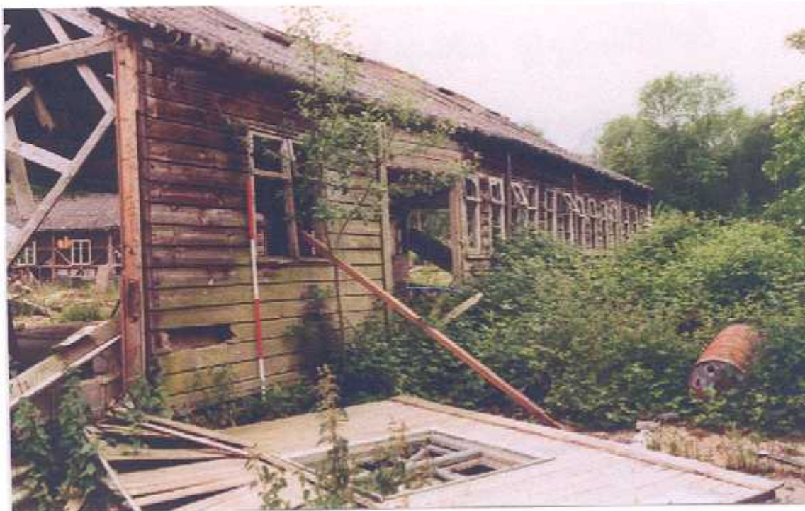
Plate 4: Structure 12 looking south. Scale 2m
