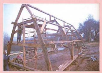
timbers of the correct size, based on the housings cut into the backs of the crucks. The original ridge had gone, so the new one is based on those surviving in similar buildings in the area.
